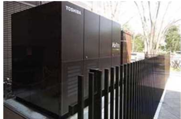
Hydrogen fuel cell power system installed at Prefectural Azuma Sports Park
