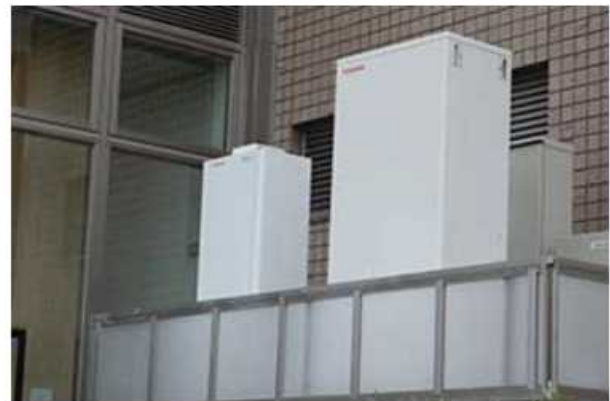
Hydrogen fuel cell power system installed at J-Village sports training facility
